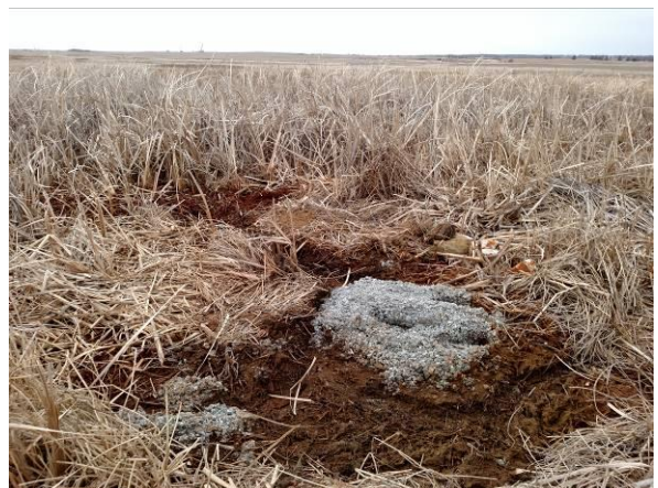
Photo #12 Sealing completion of borehole Cote 1.
