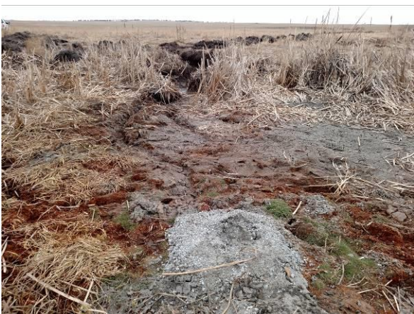
Photo #11 Sealing completion of borehole Cote 2.
