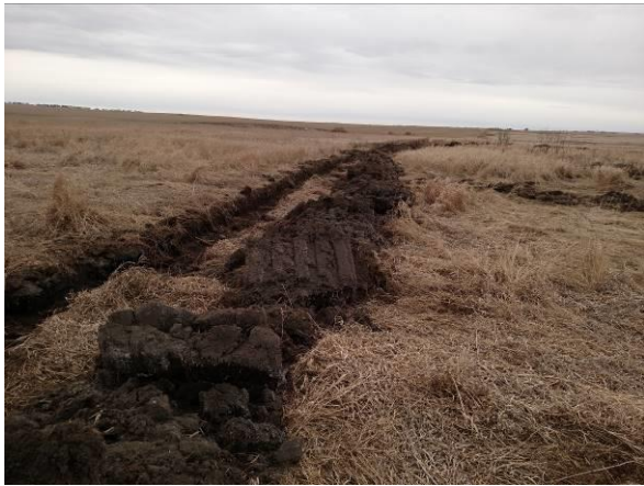
Photo #15 View of dewatering activities at borehole Cote 2.
