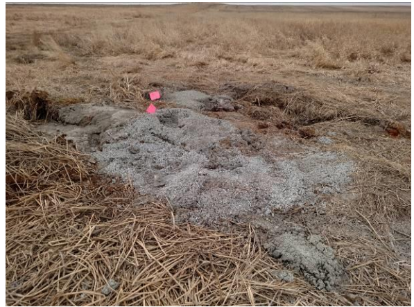
Photo #10 Sealing completion of borehole Hetzler 1.
