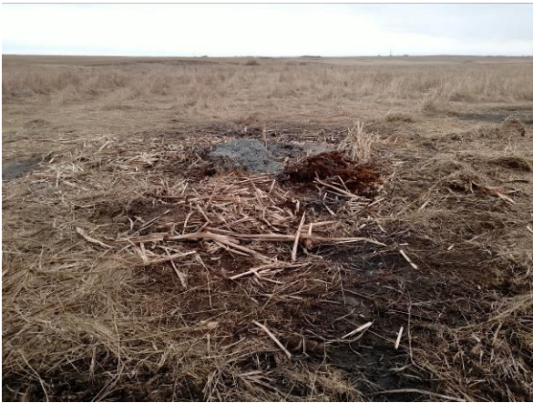
Photo #9 Sealing completion of borehole Hetzler 2.
