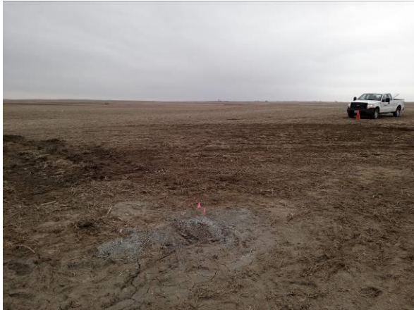
Photo #13 Sealing completion of borehole Gjorven 2.
